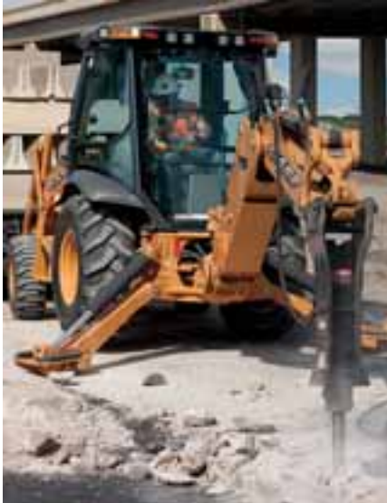
Optimized hose routing for demolition work
